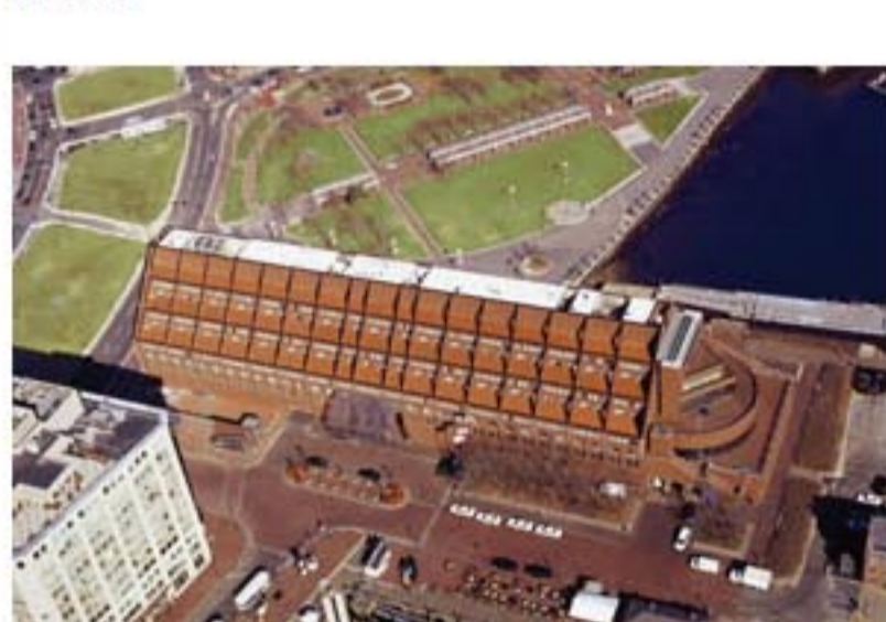
Photos courtesy of Sika Sarnafil Inc., Canton, Mass.
