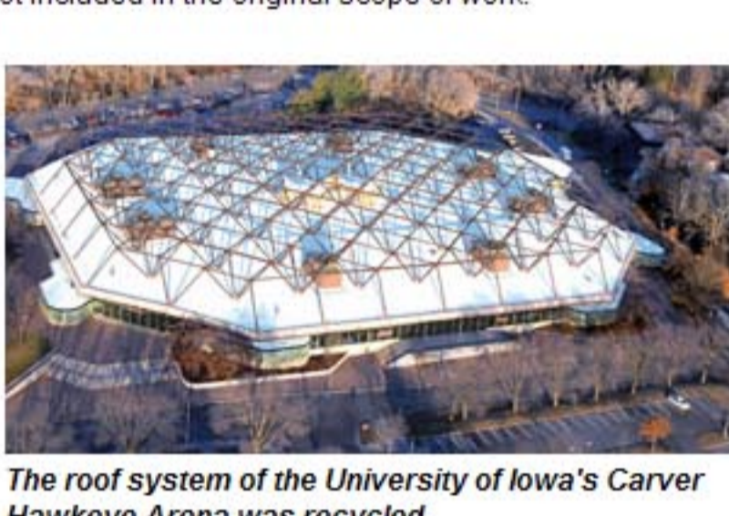
The roof system of the University of Iowa's Carver Hawkeye Arena was recycled.
