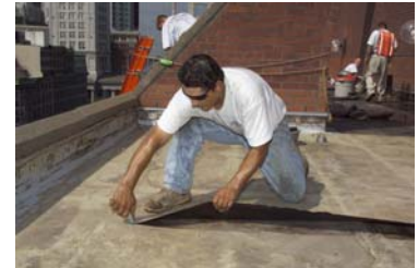
Workers remove the old membrane from the roof.
