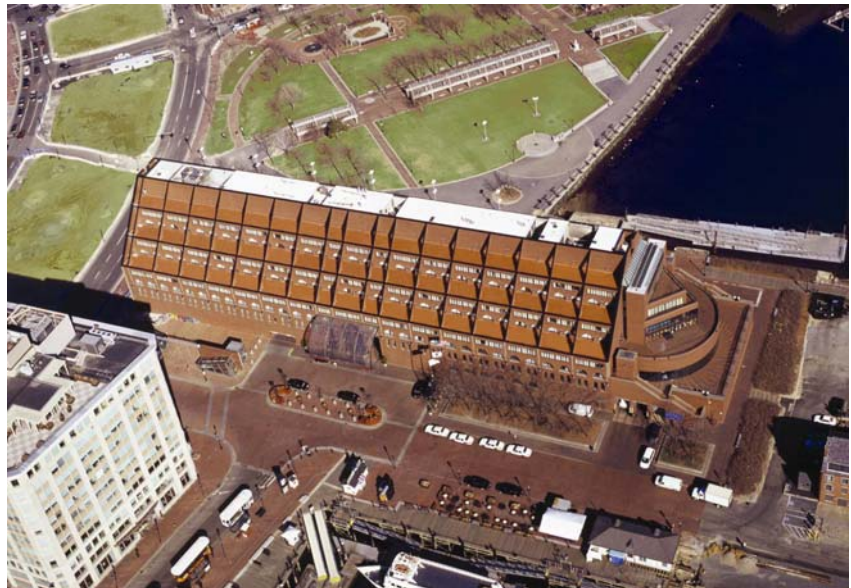
The Marriott Long Wharf in Boston, MA was one of the first in the country to have its old roof recycled into new Sarnafil material.
